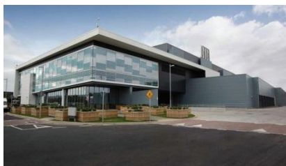
Microsoft datacenter Dublin
